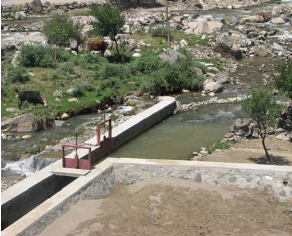
An irrigation intake, being built under the World Bank financed project in Panjsher Province.
