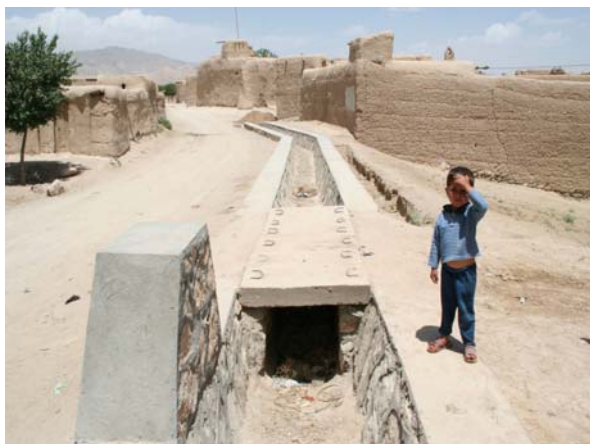
A cross drainage and culvert have been built under the National Solidarity Program in Ghazni Province.
